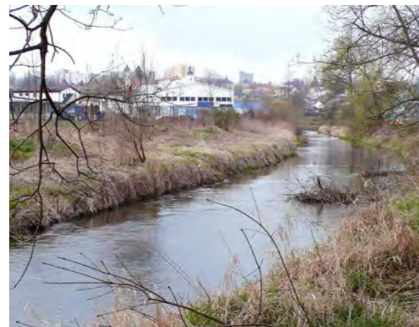
Fig. 1. Blanice river at the lower outskirts of Vlašim before revitalisation. The riverbed had geometrised technical adjustments and the banks were covered by nutrient-rich soils with ruderal vegetation. (T. Just)
