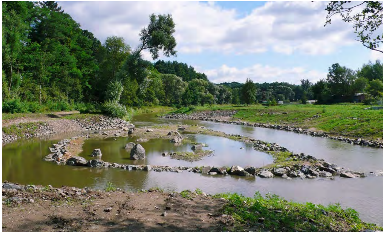
Fig. 5. There were not many opportunities to open up the Blanice riverbed in Vlašim. One of them occurred at the lower outskirts of the town. In a widened place, an untraditional islet with a pool was created. (T. Just)
