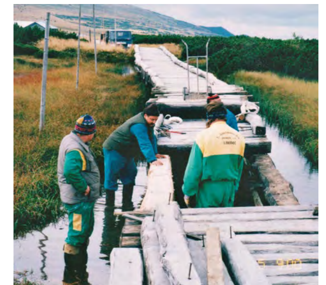
Fig. 6. Reparation of a log path through the Úpa peatbogs in 2000. (J. Harčarik)
