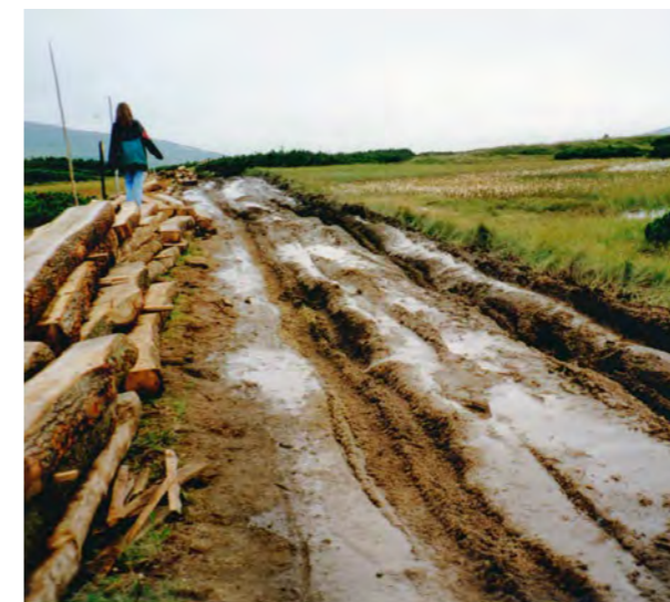
Fig. 4. Revitalisation of tourist trail through the Úpa peatbogs (removal of limestone and building of a log path) in 1996. (L. Jiříšě)
