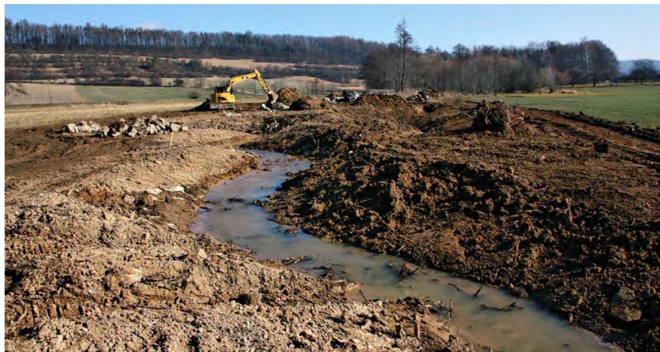
Fig. 5. In the revitalisation of the Barovka stream in the Železné hory PLA, a migration passage was created in the place where the stream flows into the Doubrava river. Already in 2015, a year after realisation, Cottus gobio was found to occur in the revitalised section. This species has a strong population in the Doubrava river, but did not occur in the stream before revitalisation. (V. Peřina)
