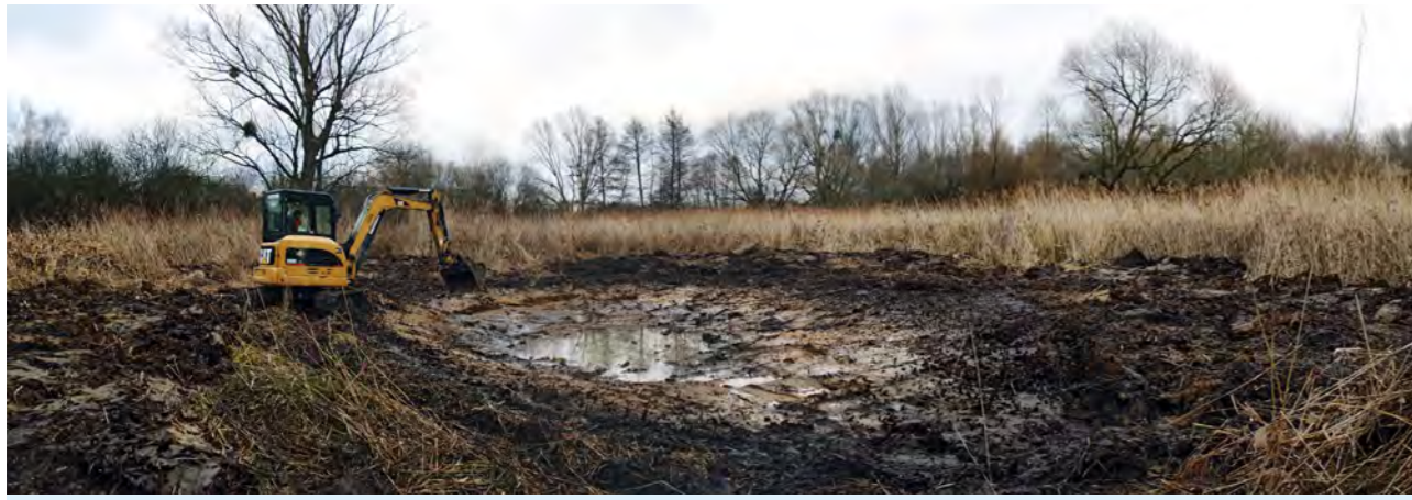
Fig. 7. In the waterlogged floodplain of the Jasénka stream near Hlučín, financed from the Landscape Management Programme, several pools of various sizes have been restored in an extensive reed bed. The aim was to increase the number of wetland habitats, which had strongly declined in the past decades by direct elimination or draining. The pools are only filled with groundwater or precipitation. Since they do not contain any fish, amphibians are provided an appropriate environment. (F. Šálek)
