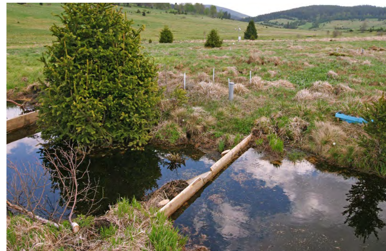
Fig. 8. Blocked draining channel after restoration. (I. Bufkova)
