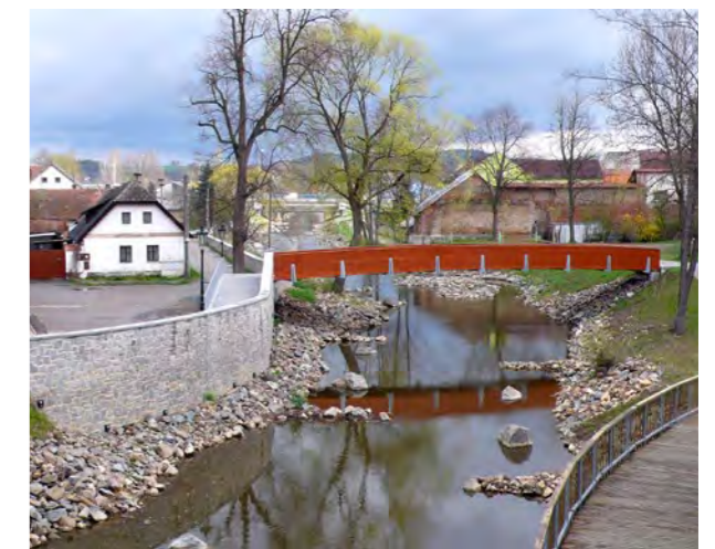
Fig. 4. Near-natural flood protection of the Blanice river in the historical centre of Vlašim. Protection walls demarcate the river corridor with a near-natural riverbed, diversified and stabilised with stone structures. New infrastructural elements – a parallel working path and bridge – are well visible. (T. Just)
